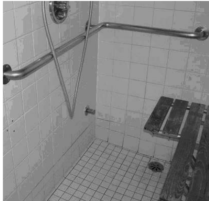
Figure 1. Steam shower seat area (outlet pipe indicated)
