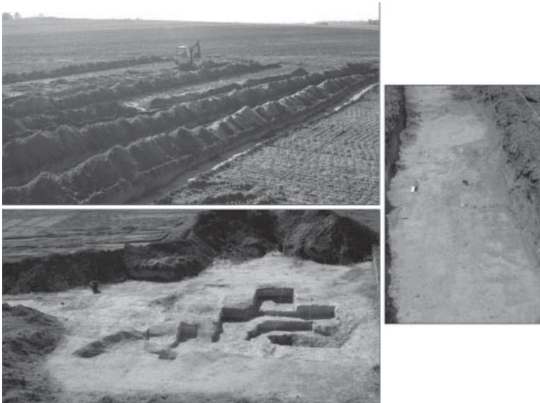
**Figure 28.4** Discovery phase and completed excavation of case study 2. Top left: trenching operations using heavy machinery to strip off the plow-zone level. Right: the first appearance of the crash crater feature in the floor of a test trench. Bottom left: completed excavation.
